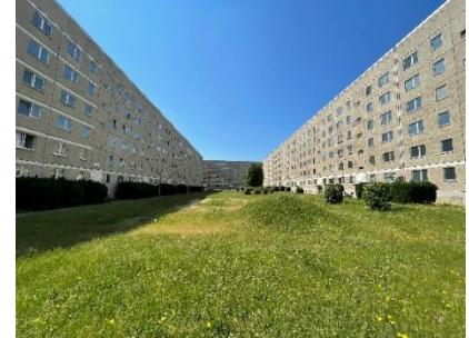
Social housing bloc in post-war neighbourhood of Altenburg; a substantial number of migrants live in neighbourhoods with a high percentage of social housing © Photo Valentin
